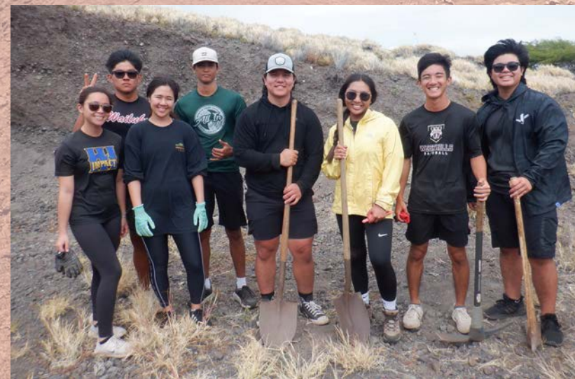
▲ Grace Bible volunteers shoveling gravel to control water on roadways in July 2023
