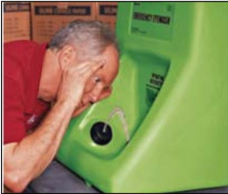
Figure 3. Portable Eye Wash Station
