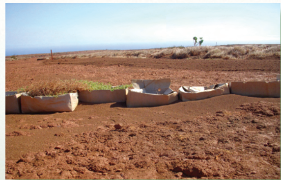
Cardboard boxes filled with wood chips capture soil and seeds
