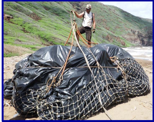
~1 ton of debris prepped and rigged for helo ops
