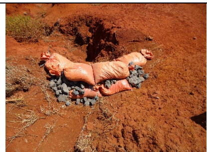
Check dam in a gully in the Project Site
