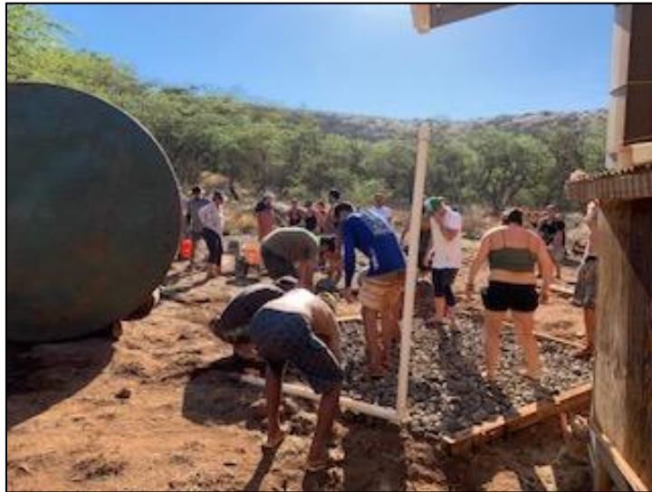
Figure 6. Leveled Out Foundation with 'Ili'ili
