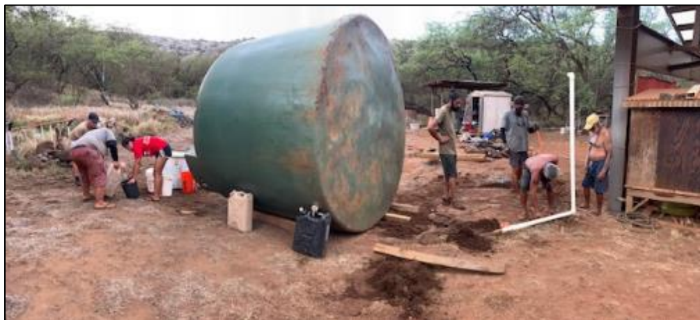
Figure 5. Water Tank Maintenance - Hawai'i Island Side
