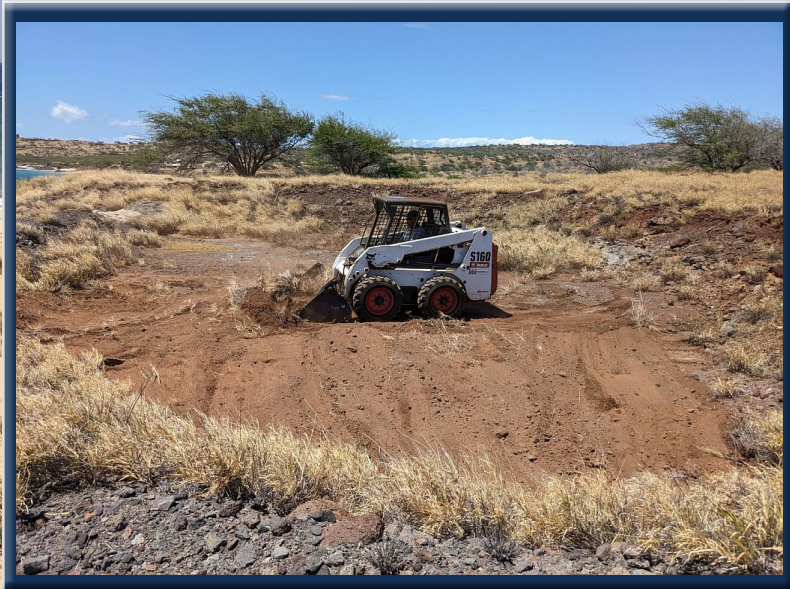
▼ Silt pond excavation in Honokanai`a in July 2023
